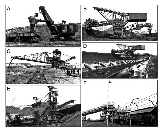
**Fig. 7.** Technological progress in the Konin Lignite Mine (KLM) during communist times. **A–C –** From single- to multi-bucket excavators and railway transport; **D–F –** Predominance of lignite and overburden transport by belt conveyors; note that on the ground surface only lignite is transported by mine railway in Figure 7F (photographs from DMK archives).
